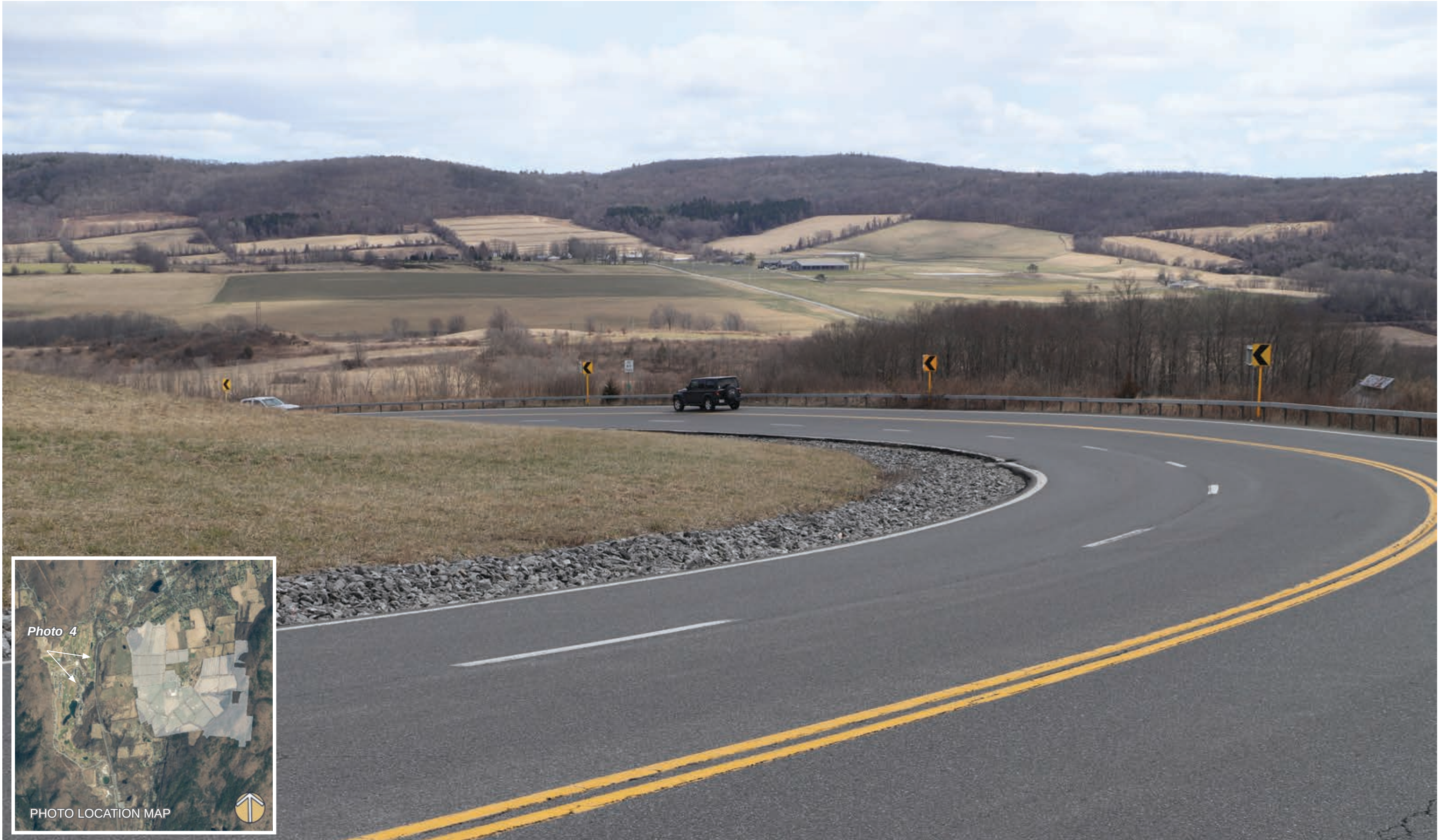
Photo 4: Route 44/W Main Street near Delavergne Hill (looking southeast) EXISTING CONDITION
