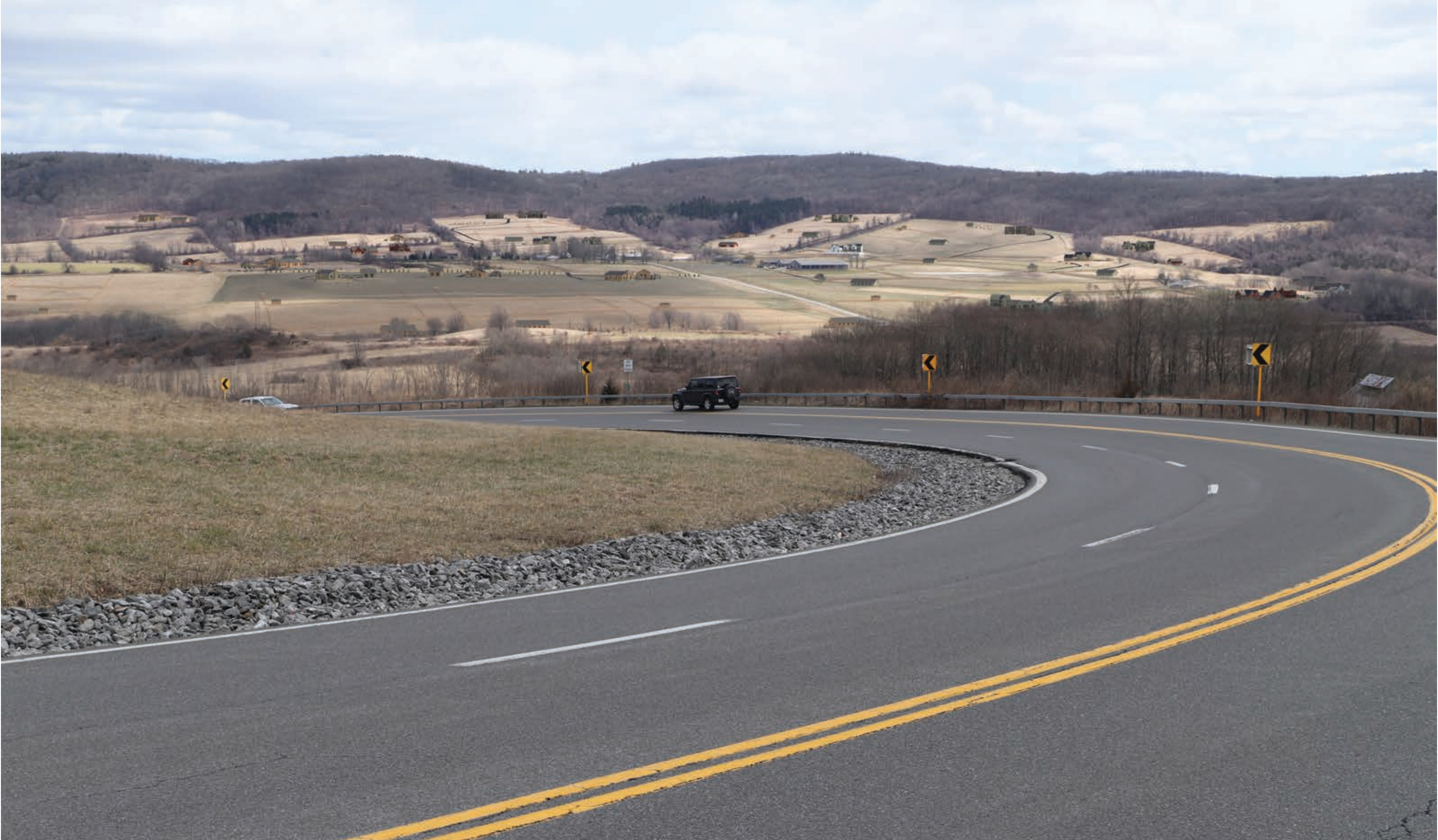
Photo 4: Route 44/W Main Street near Delavergne Hill (looking southeast) SIMULATED CONDITION
