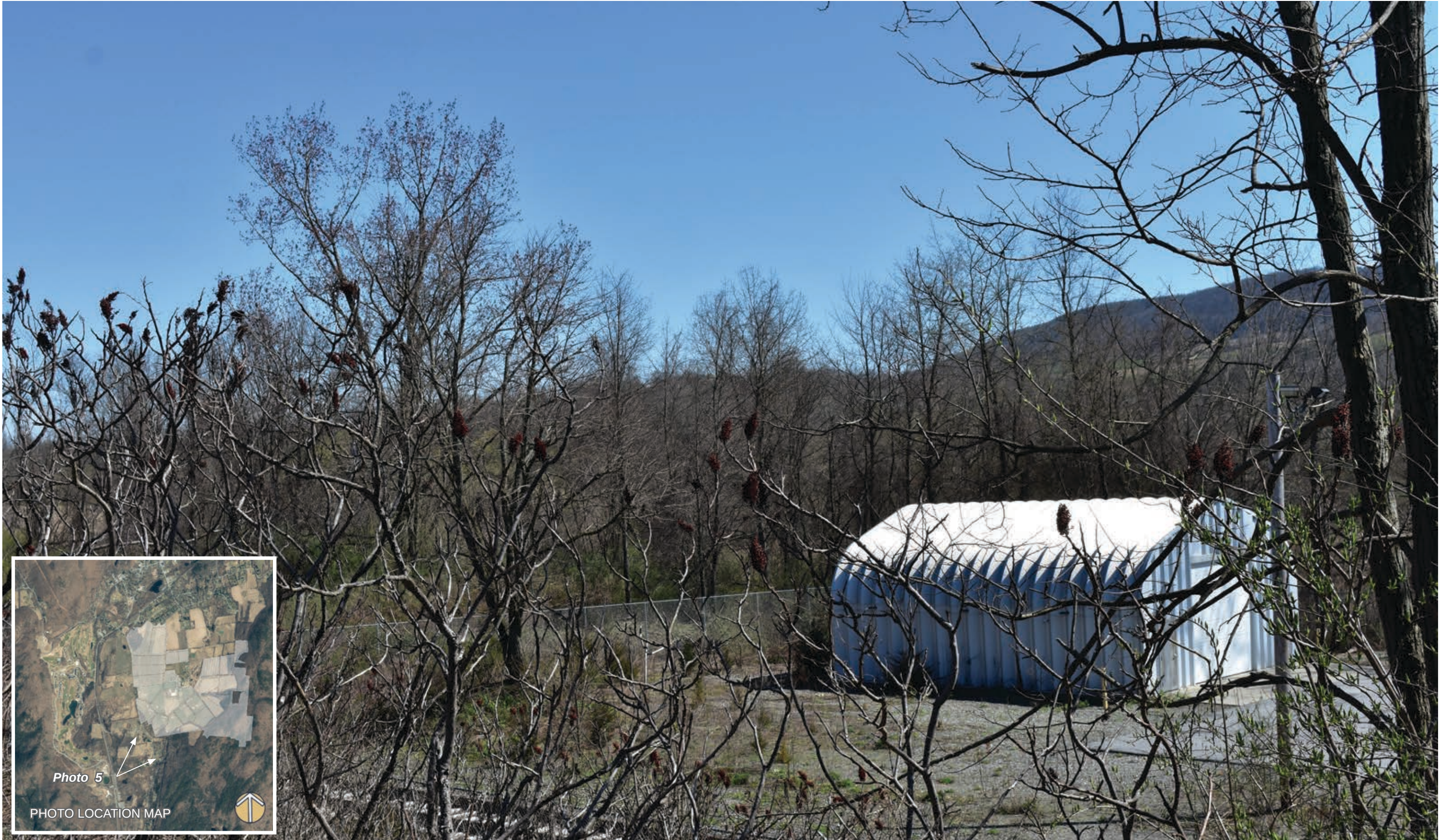
Photo 5: Route 22 north of Redtail Pass (looking northeast) EXISTING CONDITION
